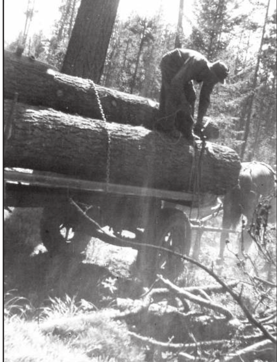
Cinching a load of logs on horse-drawn Hoover wagon
