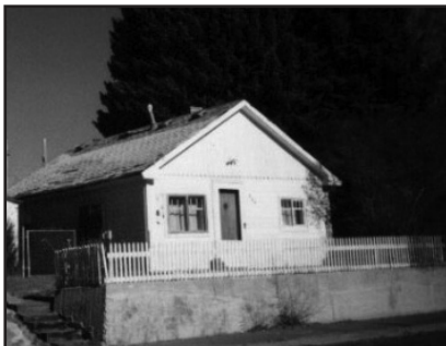
347 CLEVELAND The log cabin eventually had a concrete foundation, indoor plumbing, added room, and was covered with siding.
