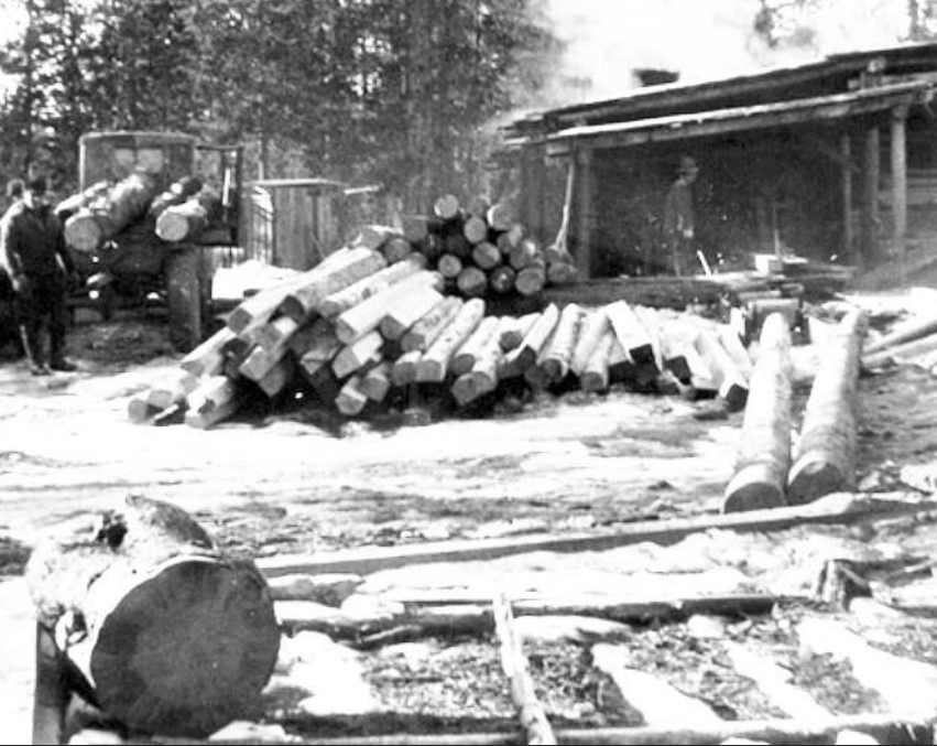
Logs loaded off the truck onto the skidway to be sawn. Logs already sawn on 3 sides ready to be loaded and shipped.
